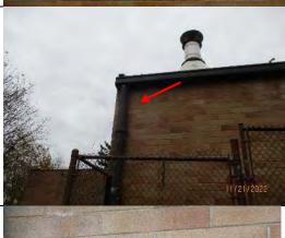
9. Closer view of previous photo showing crack through brick and mortar.
