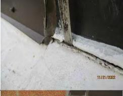
7. Sealant no longer adhered between brick and metal flashing at the base of the clerestory window at the east end of the main roof.
