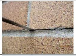
3. Overview of cracks through brisk and mortar at the north elevation below the ridge between the main roof and small roof at the northeast corner. Recommendation: Structural repair appears necessary to prevent future cracking, followed by replacement of the brick. Another option is to install new cladding, insulation, and weather barrier over the brick after structural repairs.
