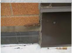
8. Unadhered perimeter sealant joints at clerestory Kalwall windows at the east end of the main roof. Recommendation: Remove existing sealant joints
