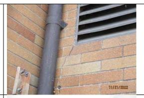
7. Damaged brick, or brick with a hole from a previous penetration at the east elevation (highlighted). Recommendation: Patch with mortar or clad over brick as indicated above.
