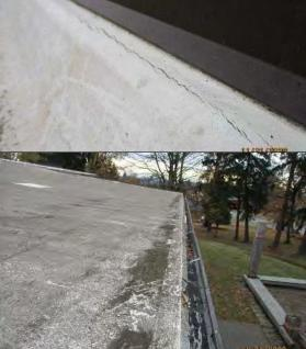
12. View of open lap joints in drip edge metal, as indicated in previous item.
