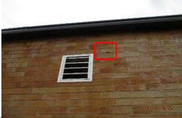
8. Cracked brick at the southeast corner, east elevation (arrow).
