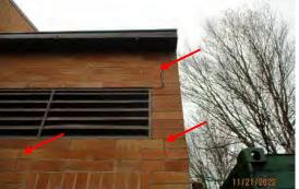
6. Additional cracks at the east elevation. *Recommendation: see previous.*
